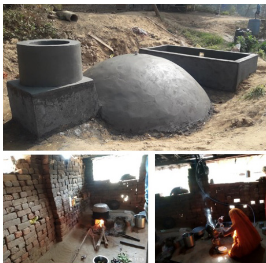
Fig. 23: Views of toilet-linked bio-gas plant, conventional chulhas and bio-gas using by beneficiary at Munjkuva village
