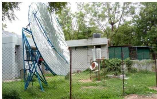
Fig. 8: Photograph of system installed at Shree Krishna Hospital (Karamsad)
