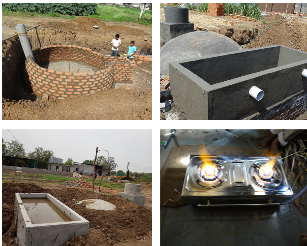
Fig. 19: View of construction of solid state bio-gas plants
