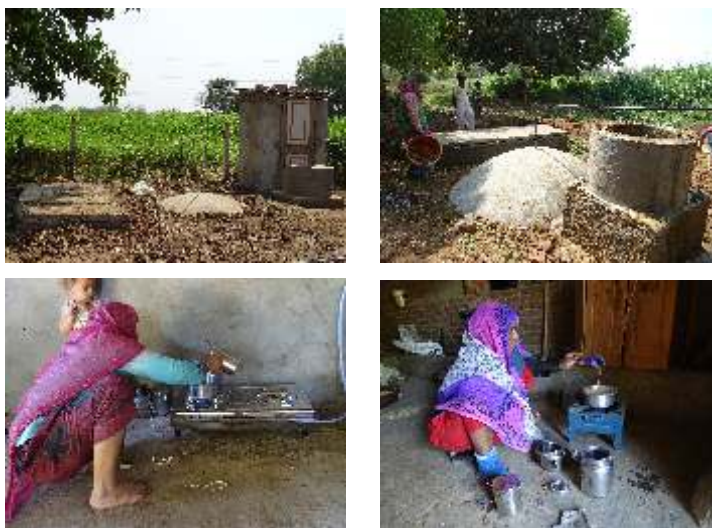
Fig. 24: Views of toilet-linked bio-gas plant and bio-gas use in kitchen
