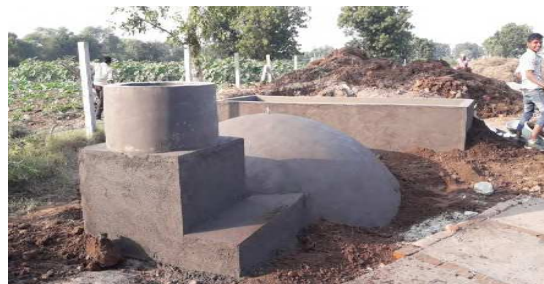
Fig. 32 Construction of solid-state bio-gas plant
