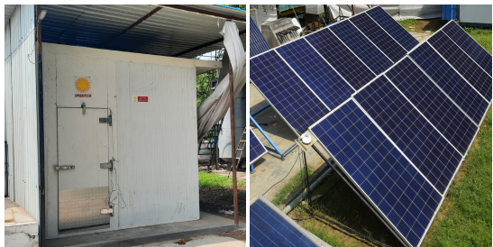
Fig.4: Installed new cold room and PV panels on the ground
