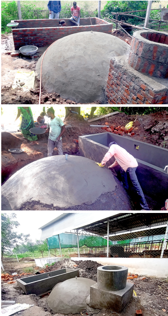
Fig. 36 Construction of solid-state biogas plant at Ajarpura, Laljipura and Shardapura village
