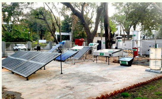
Figure 10.2: Renewable energy tech park
