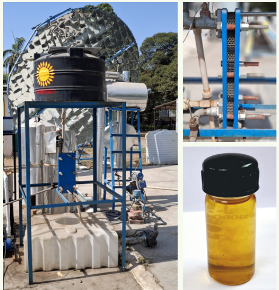
Figure 8: Scheffler reflector based essential oil extraction system
